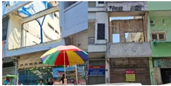
Figure 5. Waroeng Hill: Demolished Building
