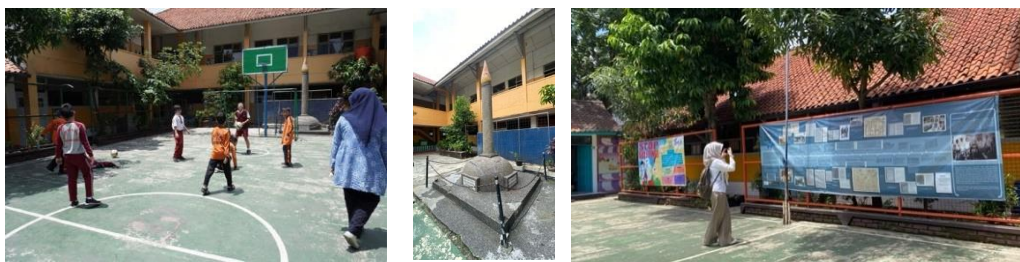
Figure 2. Exterior Condition of Living Museum Building
