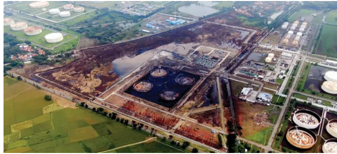
Figure 4. Areas Affected by Fire
